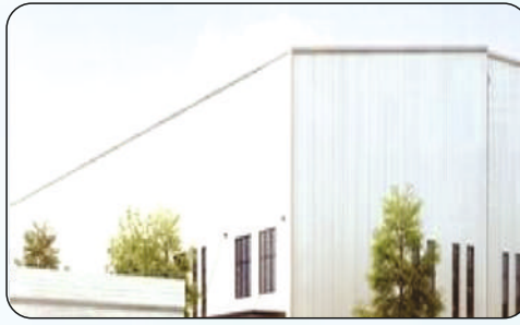
Project Name : ATL Battery Location : BAWAL, Haryana
