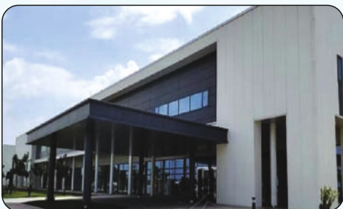
Project Name : Oppo Mobile Location : Noida, UP
