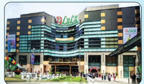
Project Name : Lulu Mall Location : Lucknow
